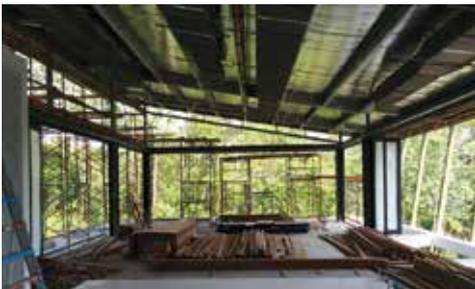
For the mono-pitch roof to work successfully it has to extend far enough from the face of building. (Rantau Panjang House by SML Architects.)
