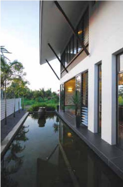
The roof eaves are extended lower on the west facing side of this house. (1-tree House by Design Network Architects.)
